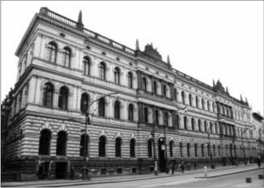
Fig. 5 - Building of the Academy of Sciences of the Czech Republic
